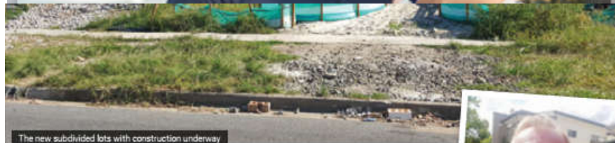
The new subdivided lots with construction underway
